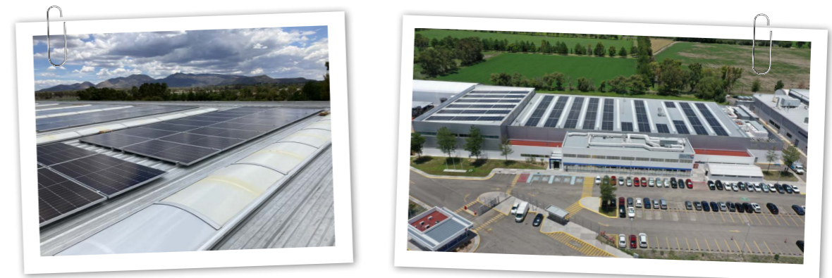
Our photovoltaic system in Mexico after its implementation in August 2022
